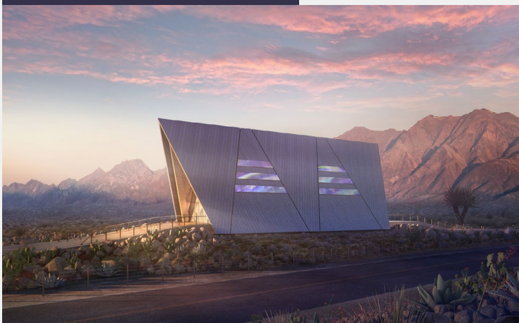
Oklo's Aurora Powerhouse
